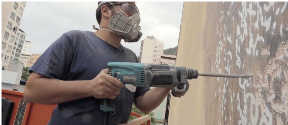
Excavation Process in 2013
