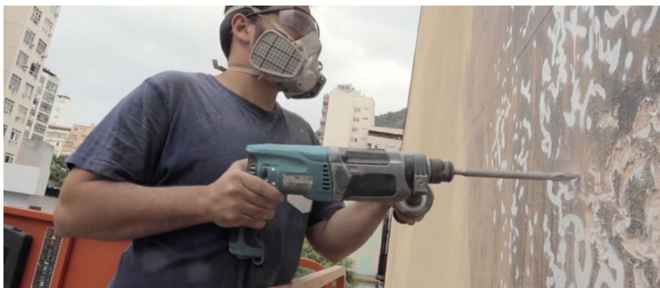
Excavation Process in 2013
