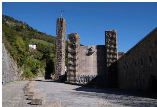
Figure 1. Picture of the current sanctuary’s front view.
